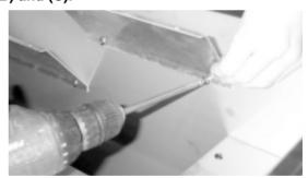
G. Unscrew the screws on the duct panel and pull it out as the picture below.
