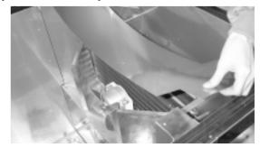
H. Unscrew the screws on the duct panels in front of the evaporator.
