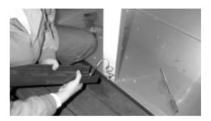
C. Disconnect the mullion heater and pull out the mullion insulator.
