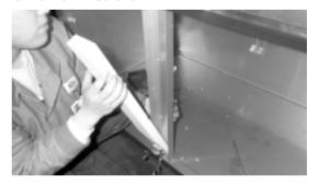
D. Unscrew the screws on top and bottom of the mullion. Replace the old one with new.
